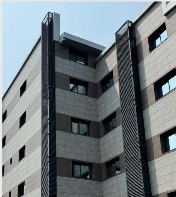
Africa, Gabon Office building
