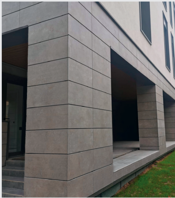
Spain, Pamplona Residential building
